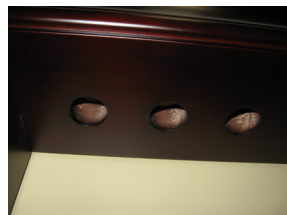
Top hole detail - Eight 1" dia. holes evenly spaced approx. 1.125" apart w/ 1.25" space at back & 2" in front, 1.375" space at sides before holes start
